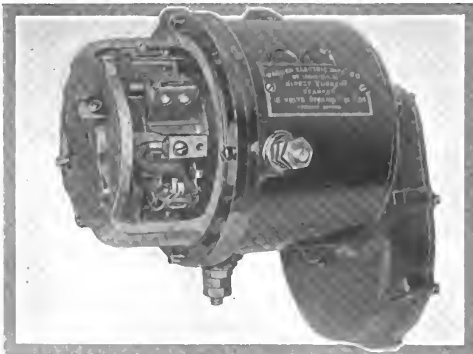
Wagner direct current starter used on 1915 Studebaker
